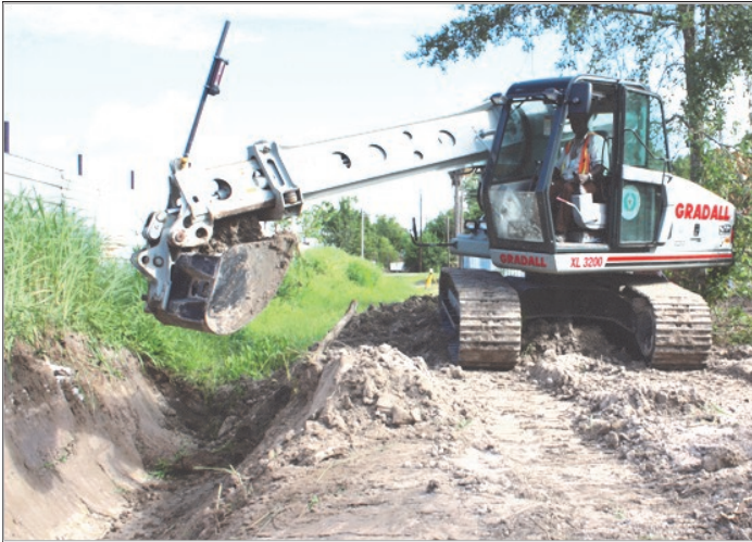
Precinct One's Jerry Lee clears dirt from a ditch on East Mount Houston to improve drainage in the northeast Harris County area.
